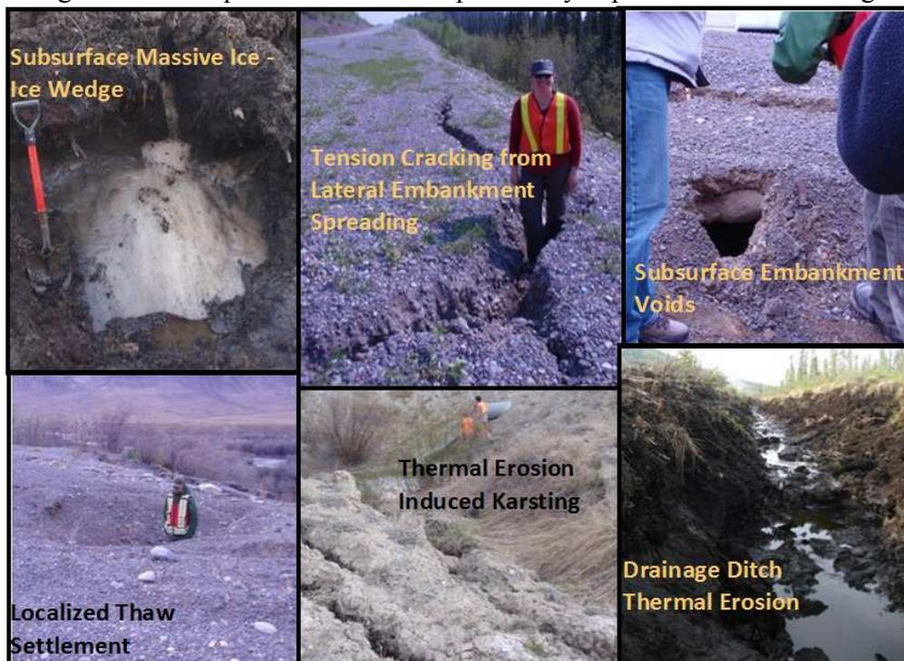
Figure 1. A collection of photographs showing the possible failure modes of a roadway on permafrost taken by the author in Summer 2014 on the Alaska and Dempster Hwys, Yukon Territory, Canada.
