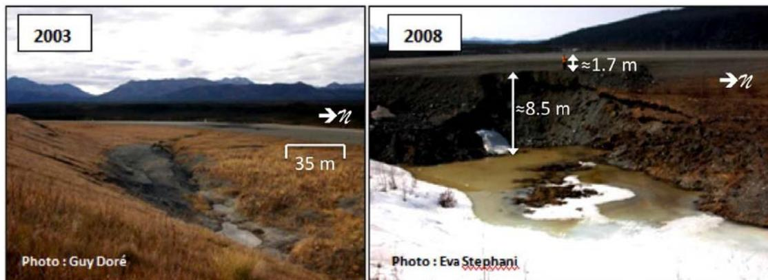
Figure 2. Evolution (2003-2008) of settlement on the east side of the road, Dry Creek rest area (location 2 in Figure 1). Left: linear depression incised in gravel at the foot of the revegetated borrow pit. The highway embankment is in the background. Right: large depression at the base of the road embankment (person for scale).
