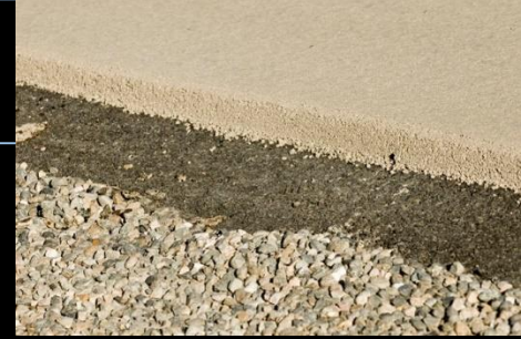
Dawson City Front Street, Yukon (Colas)
