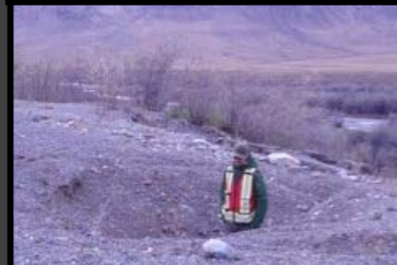
Localized Thaw Settlement
